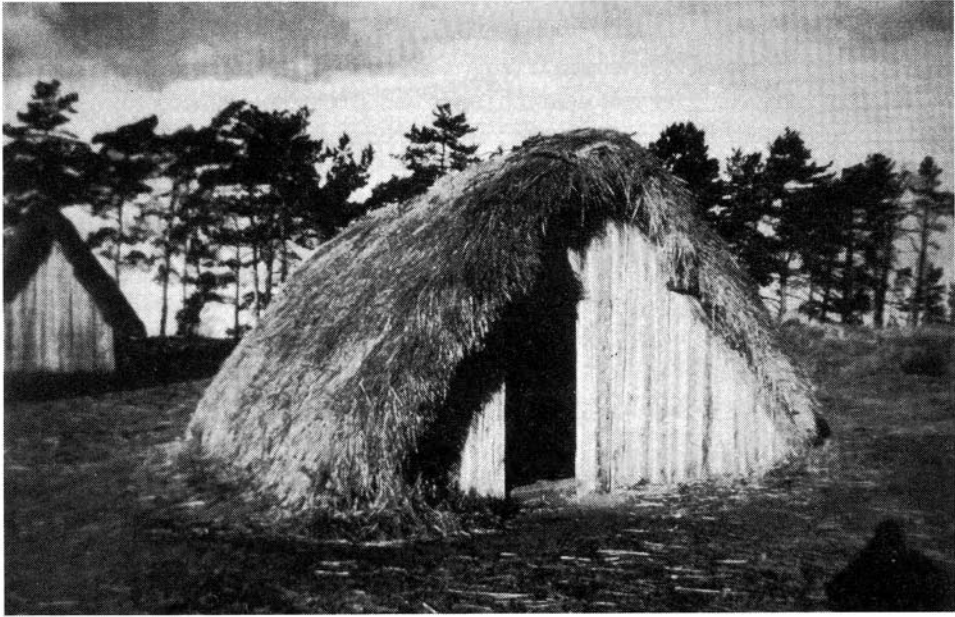
Fig. 1. Reconstructed Anglo Saxon building at West Stow, Suffolk.
